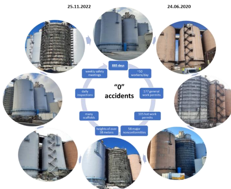
Fig. 12. The evolution of the consolidation of the phosphate silo
