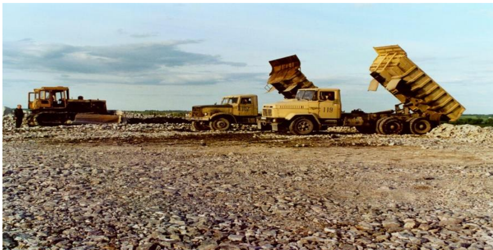
Fig. 4. Mining and technical reclamation of the tailings storage facility in the quarry of brown iron ore (photo, Zhovti Vody, Ukraine)
